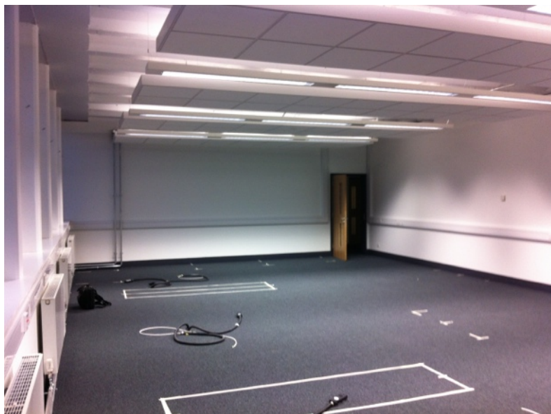
Fig. 3 Whilst the lighting for this office space may be designed to reduce potential glare on display screens, the lit effect in the room is very poorly considered. A very dark end wall and messy spill light of the side wall do nothing to inspire confidence that the installers cared about the end users of the room. As a student project, a similar space was dramatically improved by removing all the complicated optics from the fluorescent luminaire and adding a vaulted soffit of white card above the luminaires to capture and diffuse the uplight component.
