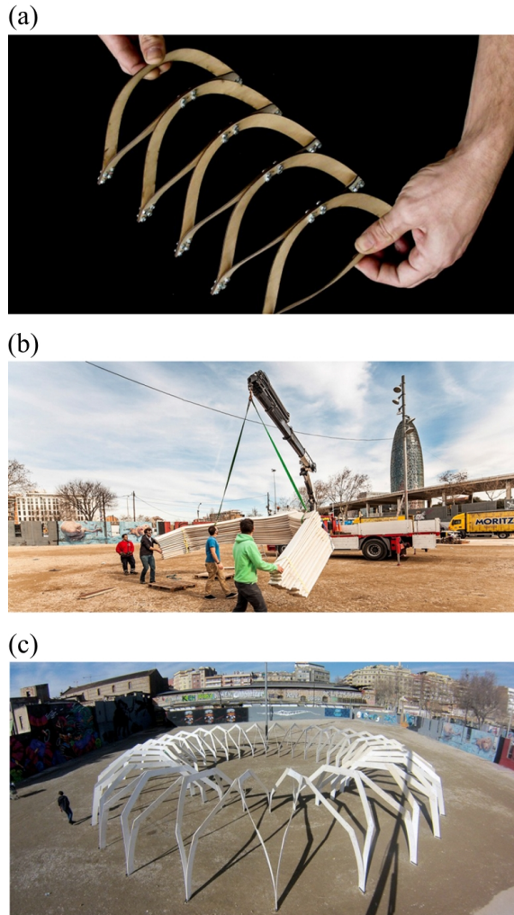
Figure 2: Pliable timber torus pavilion, Barcelona, 2014 [17], by: CODA (Computational Design Affairs): (a) Model prototype; (b) Construction phase; (c) Realised structure. Photos courtesy: David S. Anderson (WIT Press).
