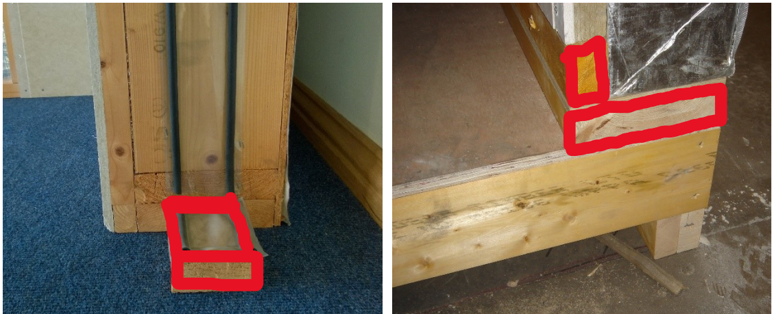
Figure 3-14 Sole plate detail for closed panel (in red)
