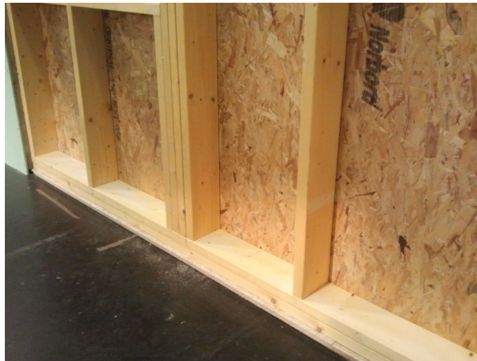
Figure 3-13 External open panel timber frame wall
