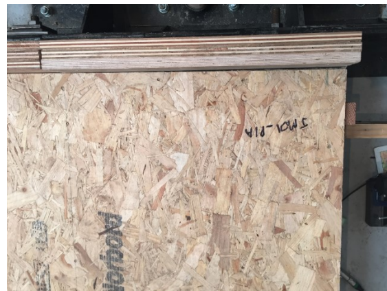
Failure observed in P18
