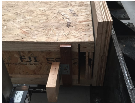
Failure observed in P17
